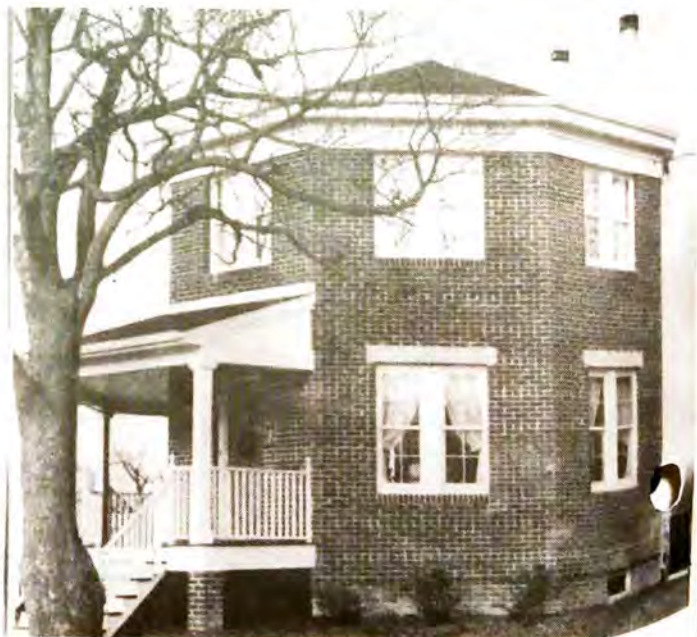
Figure 7. 26 Church Street, Belford
