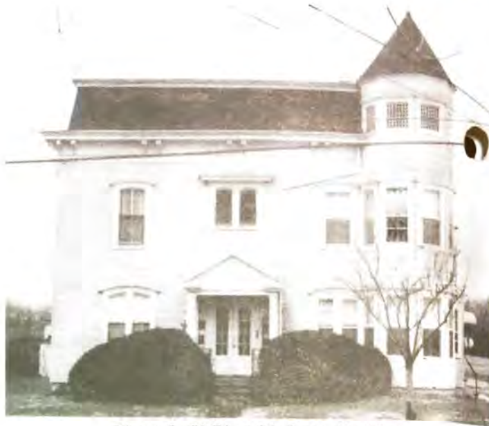
Figure 5. 59 Riverside Drive, Red Bank
