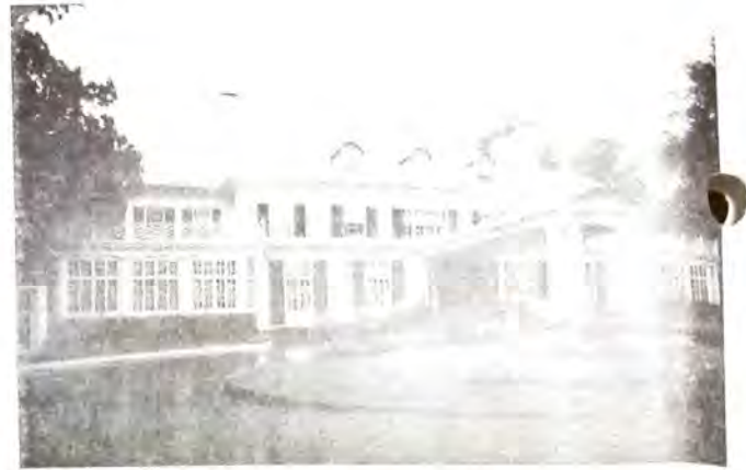
Figure 19. The Dr. Ernest Fahnestock house as a restaurant. The canopy was a later addition and side porches were enclosed.
