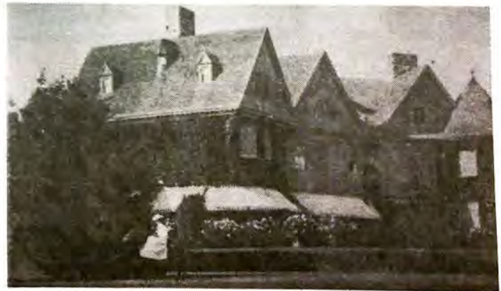
Figure 11. Rohallion, Bellevue Avenue, Rumson, before remodeling.
