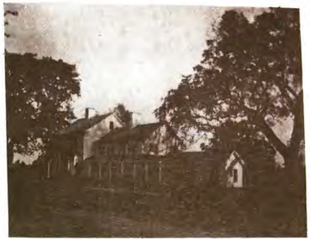
Superintendents residence - after remodeling
