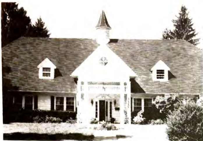
Carriage house - as residence
